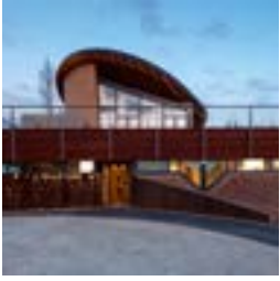
Maggie's Newcastle (designed by Ted Cullinan of Cullinan Studio Architects, landscaping by Sarah Price), in the grounds of the Freeman Hospital, Newcastle upon Tyne, opened in May 2013.
