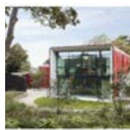
Maggie's at The Royal Marsden at the Zoë and Andrew Law Building (designed by Ab Rogers of Ab Rogers Design, landscaping by Piet Oudolf) in the grounds of The Royal Marsden Hospital, Sutton, opened in October 2019.
